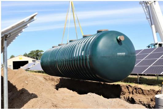
To fit into this innovative system, Panelview needed a tank that could be easily customized to serve multiple functions. It also had to be easy to deliver and install in a tight excavation footprint, which was between two rows of solar panels. Beyond that, the installation process had to be easy and straightforward since Madison was installing it himself. Our lightweight corrosion-resistant tank met these needs.
